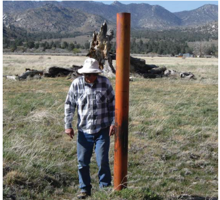
Above, an open irrigation system ventilation pipe. Below, carcasses and bones of birds and other wildlife that collected at the bottom of an open pipe (photo by Jeff King).
